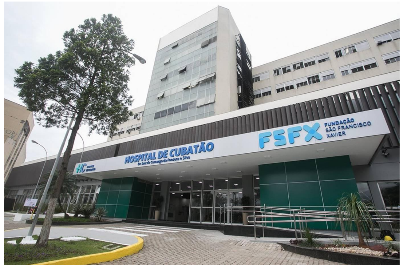
Hospital Municipal de Cubatão
